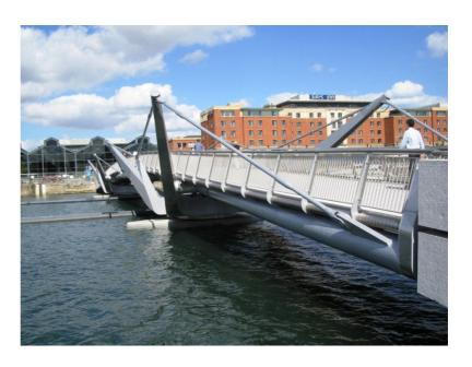
The pedestrian bridge over the river Liffey in Dublin runs approximately 100 metres in length, pivoting about the centre axis to allow river traffic to pass. CANAL produced sleek and practical light box design with a 'shot peened' finish lining the sides of the bridge. CANAL also supplied the elliptical handrails which again were complemented with a shot peened finish to overall create this prestigious project.
